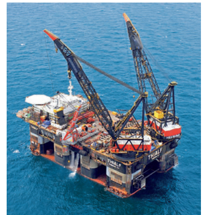
西门子能源变压器应用在深海钻井平台 Siemens Energy transformer in deepwater drilling platform.
